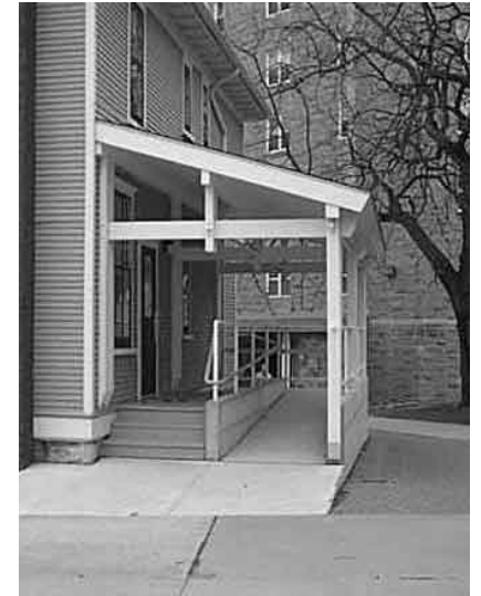
Stepped entry with integrated wheelchair ramp
